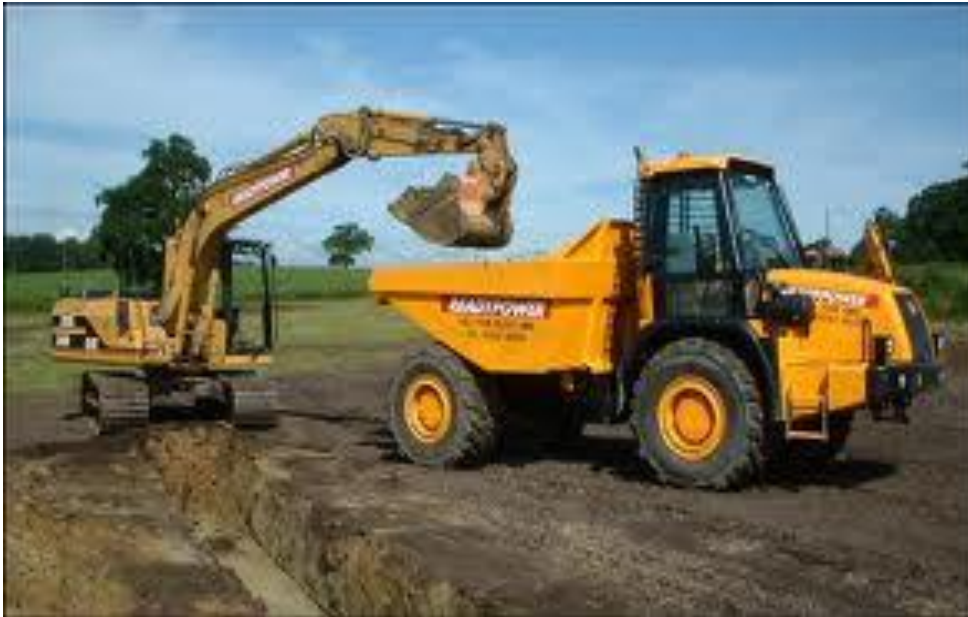
EXCAVATOR AND DUMP TRUCK
